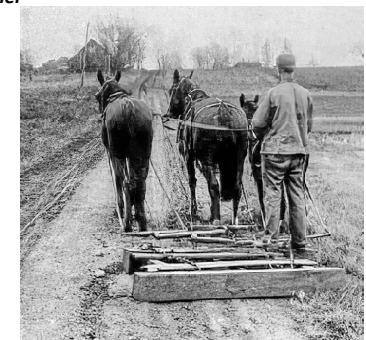
Maintenance of dirt roads, was done infrequently using primitive log "drags"
