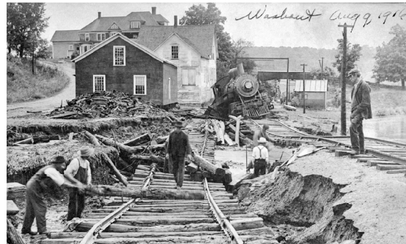
On August 9, 1916, the Tomifobia River overflowed its banks and washed out the railroad tracks at Smith's Mills (Tomifobia). Image courtesy of Stanstead Historical Society.
